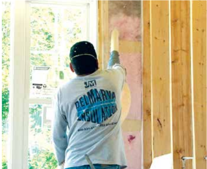
R-23 BLOWN-IN INSULATION
