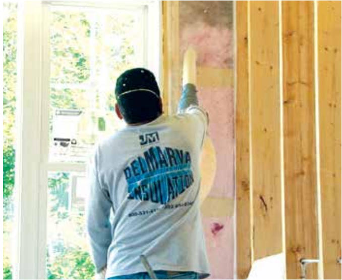
R-23 BLOWN-IN INSULATION
