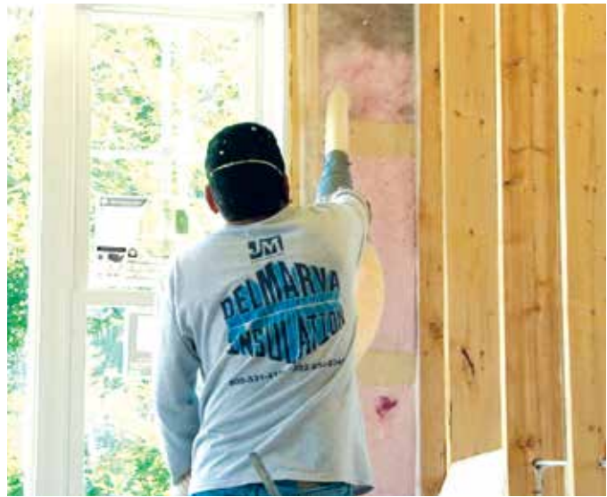
R-23 BLOWN-IN INSULATION
