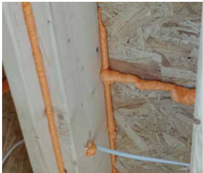
ENERGY STAR DRAFT STOPPING
