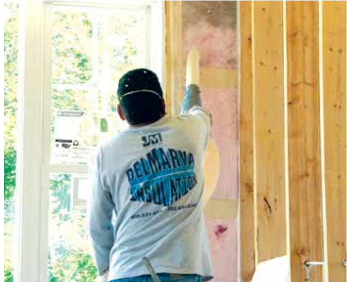
R-23 BLOWN-IN INSULATION
