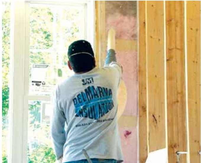
R-23 BLOWN-IN INSULATION
