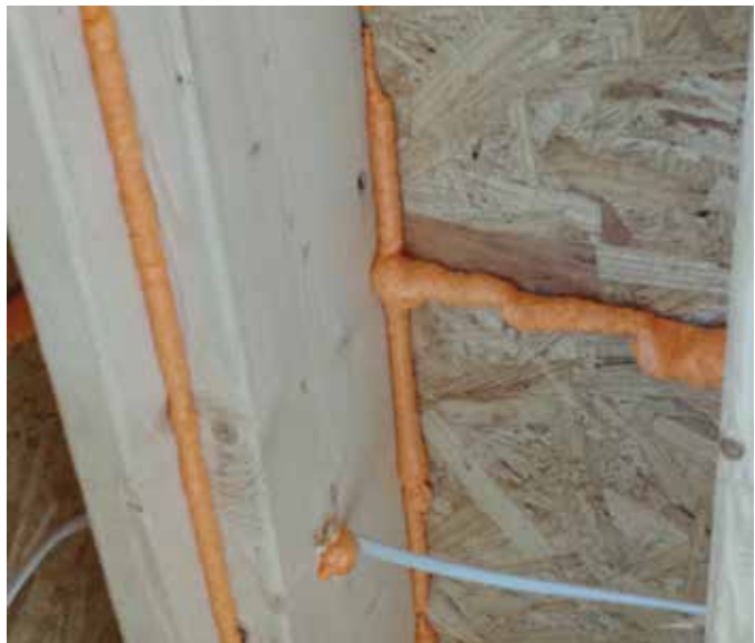
ENERGY STAR DRAFT STOPPING
