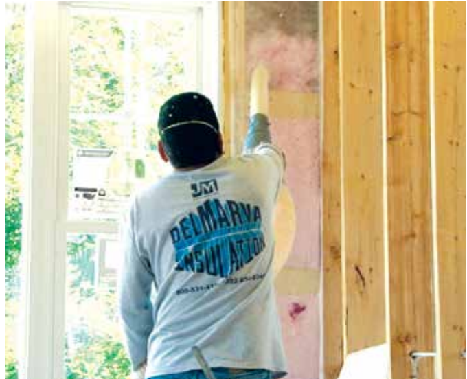
R-23 BLOWN-IN INSULATION
