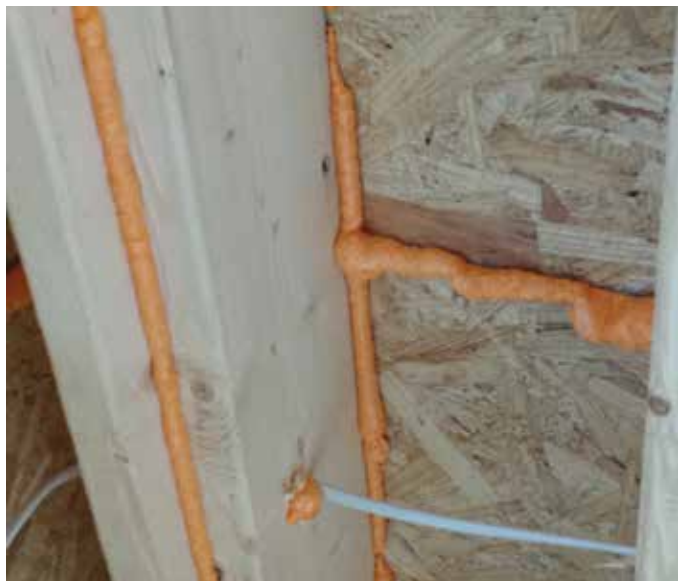
ENERGY STAR DRAFT STOPPING
