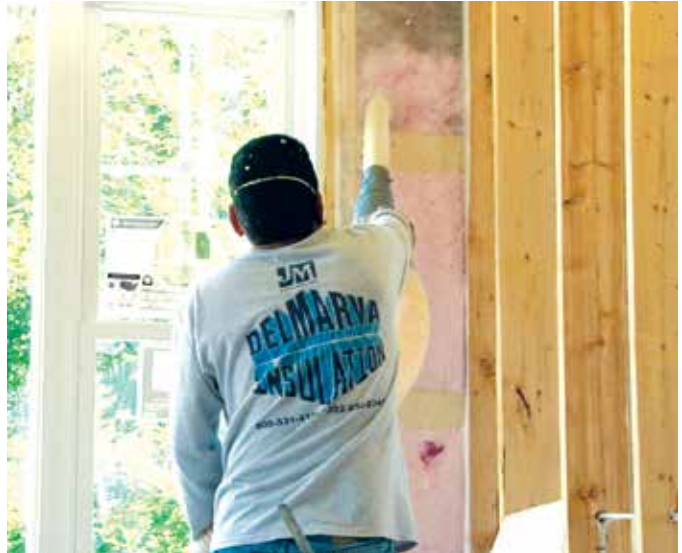
R-23 BLOWN-IN INSULATION
