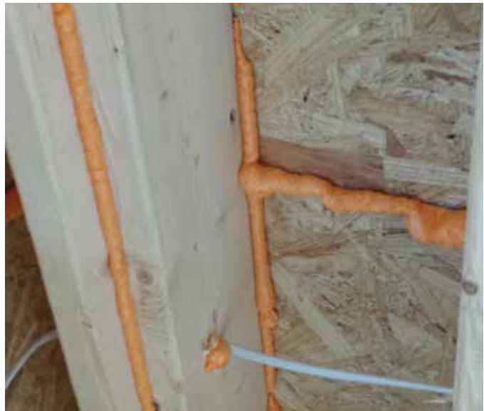
ENERGY STAR DRAFT STOPPING
