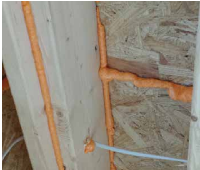
ENERGY STAR DRAFT STOPPING
