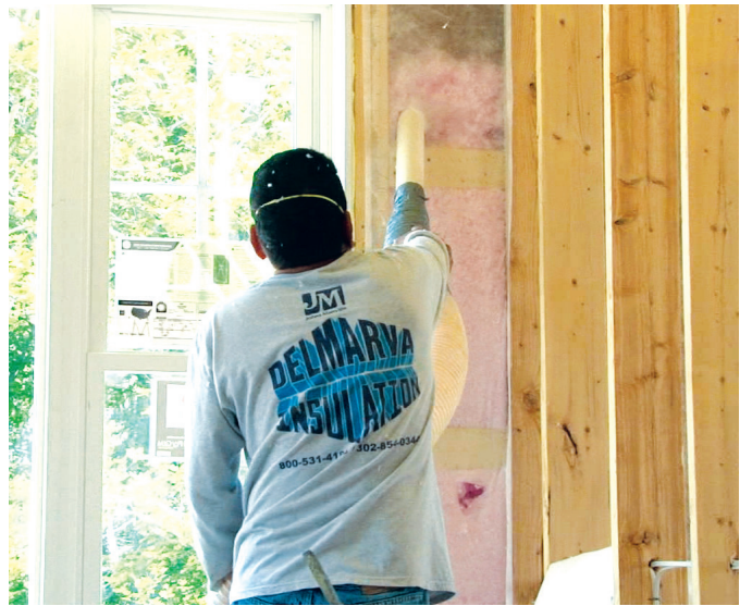
R-23 BLOWN-IN INSULATION
