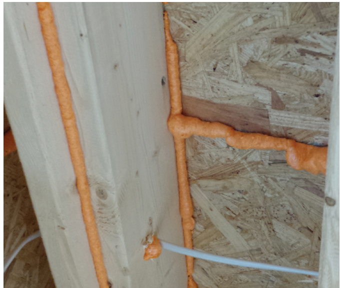
ENERGY STAR DRAFT STOPPING
