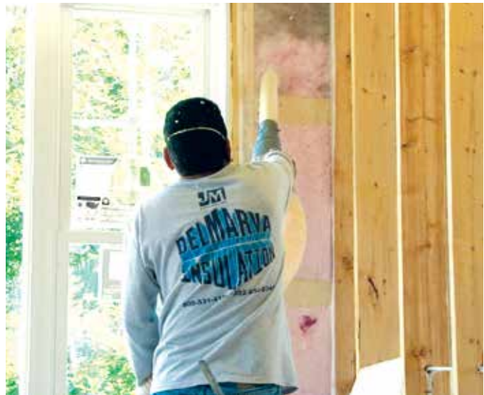
R-23 BLOWN-IN INSULATION
