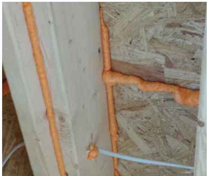
ENERGY STAR DRAFT STOPPING
