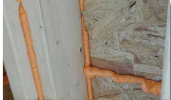
Energy Star Draft Stopping
