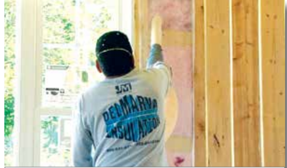
R-23 Blown-in Insulation
